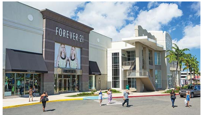
We invested approximately $540 million in redevelopment projects in 2012. Projects completed include Above: the redevelopment of Plaza Carolina in Carolina (San Juan), PR
